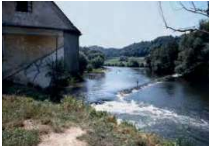
A small dam
