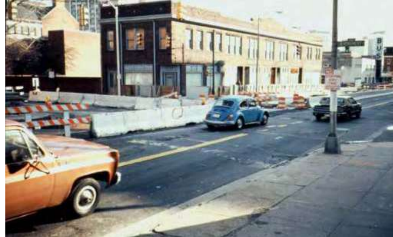
Promenade construction in process
