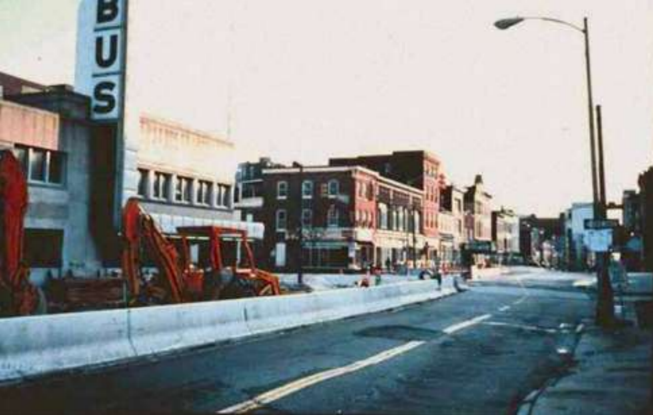
Howard Street construction in process
